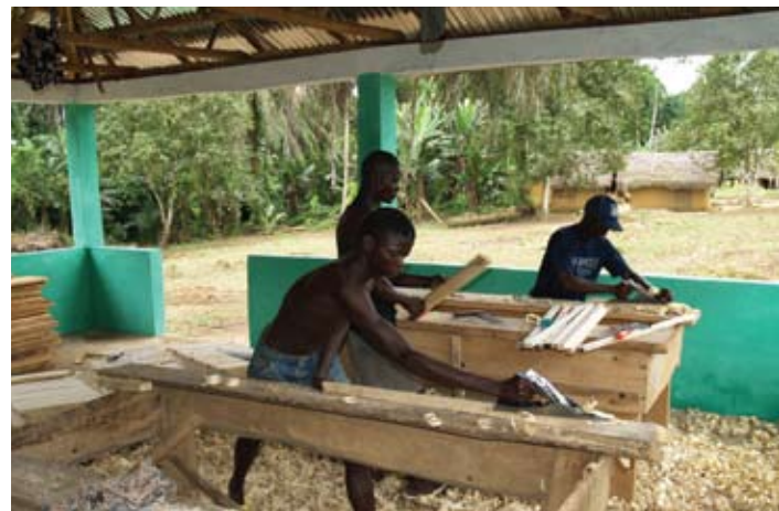
Carpentry workshop, Sierra Leone
